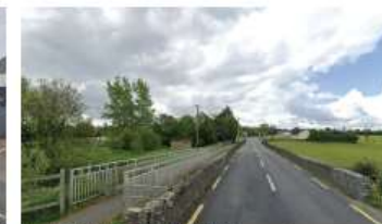
8 Johnstown Bridge at County Boundary
