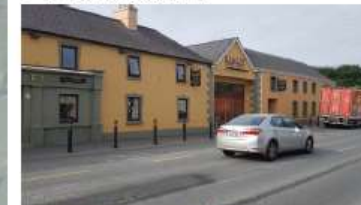
3 Main Street from Johnstown Road Junction
